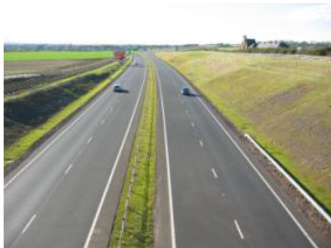
Carriageways, image courtesy of Atkins
